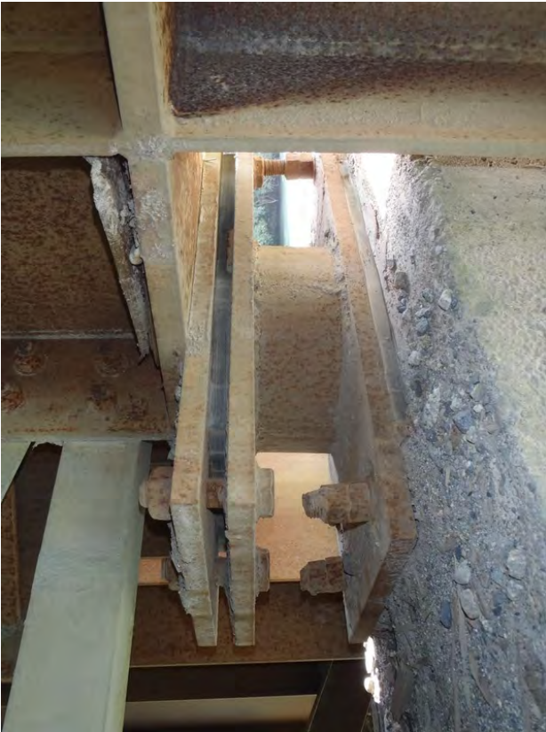
Figure 30: Typical bearing condition, Pier 2 Span 3 downstream bearing shown.
