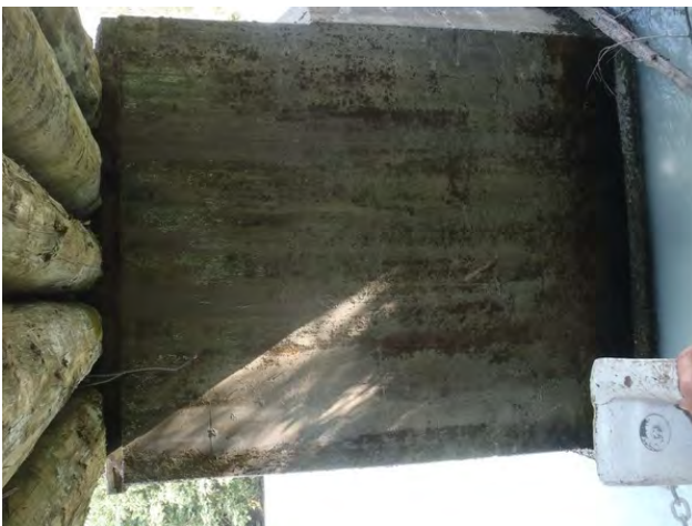
Figure 17: Pier 1 left end face.
