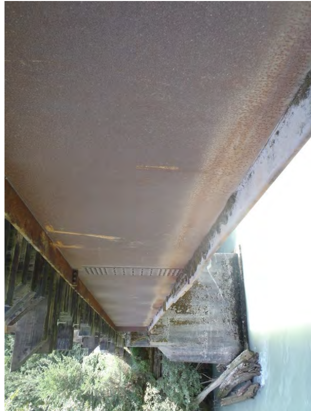
Figure 28: Typical condition of exterior face of steel girders, Span 2 Girder 1 shown.
