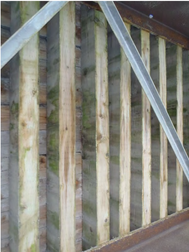
Figure 13: Typical underside of deck, Span 3 shown.
