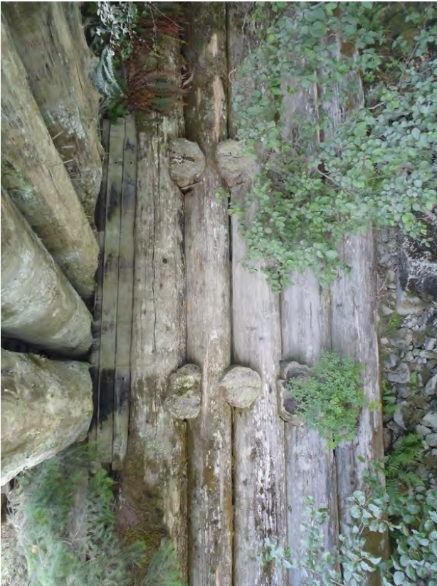
Figure 14: Left end abutment.
