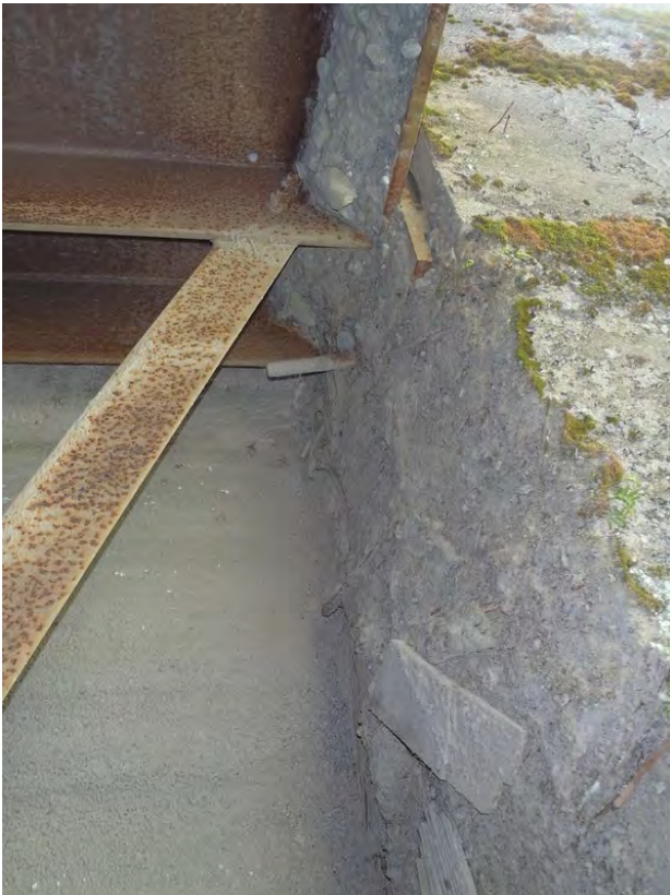
Figure 25: Debris accumulation on Pier 1.
