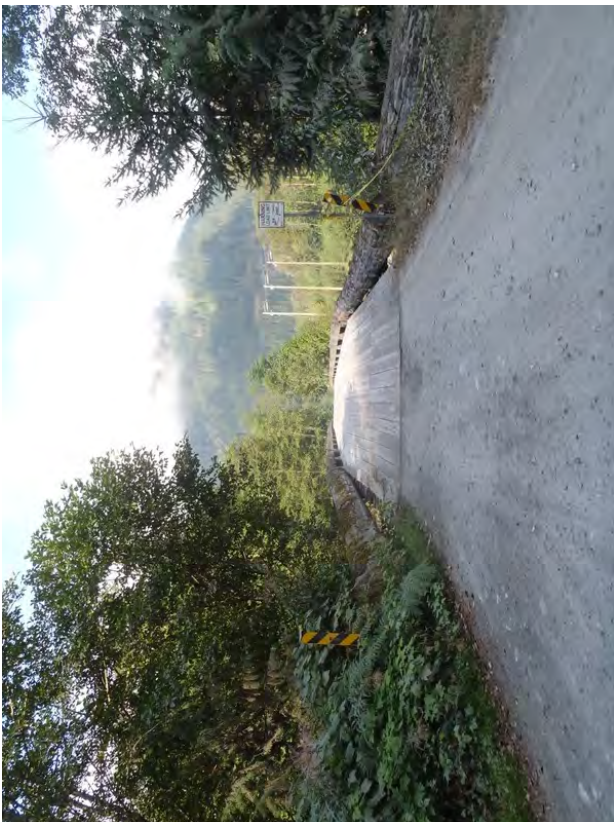
Figure 5: Left end approach.
