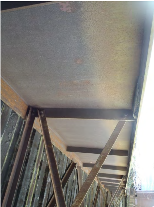
Figure 29: Typical condition of interior face of steel girders, Span 2 shown Girder 1 shown.
