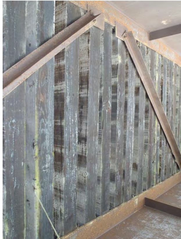
Figure 12: Typical underside of deck, Span 2 shown.
